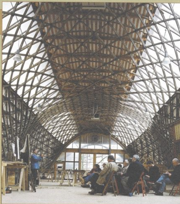
Above: 'Downland Gridshell', Weald and Downland Museum, Sussex, United Kingdom, 2002. Architect: Edward Cullinan Architects. Image © Richard Learoyd. One of three projects in the group Evolving Ideas which showed how central the collaboration of architect, engineer and maker is to the process of designing innovative buildings.
