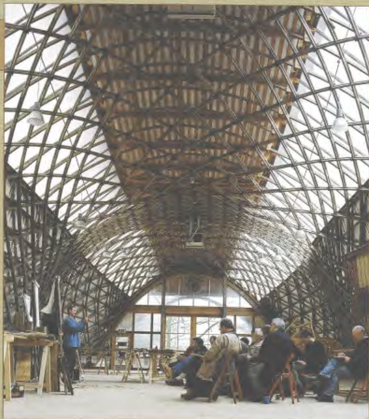
Above: 'Downland Gridshell', Weald and Downland Museum, Sussex, United Kingdom, 2002. Architect: Edward Cullinan Architects. Image © Richard Learoyd. One of three projects in the group Evolving Ideas which showed how central the collaboration of architect, engineer and maker is to the process of designing innovative buildings.
