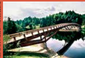
03 The Bridge at Kjearra, Lardal, Norway 2001. Architect: Arne Eggen
