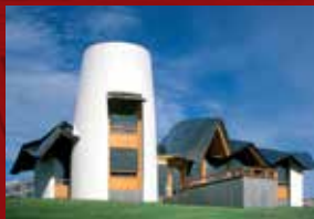
01 Maggie's Centre, Dundee, Scotland 2003. Architect: Frank Gehry
