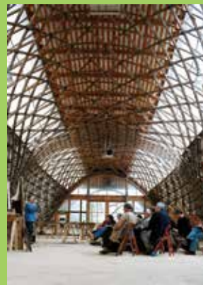
01 Downland Gridshell, built in 2002 for the Weald and Downland Open Air Museum. Edward Cullinan Architects
