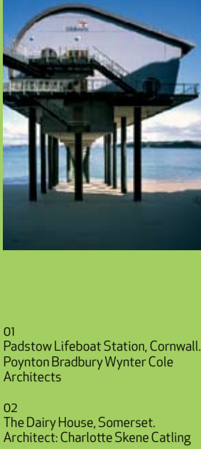
01 Padstow Lifeboat Station, Cornwall. Poynton Bradbury Wynter Cole Architects
