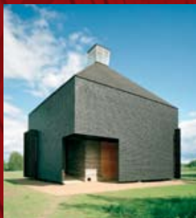
02 Wooden Church of Kårsämäki, Finland 2004. Architects: Lassila Hirvilammi
